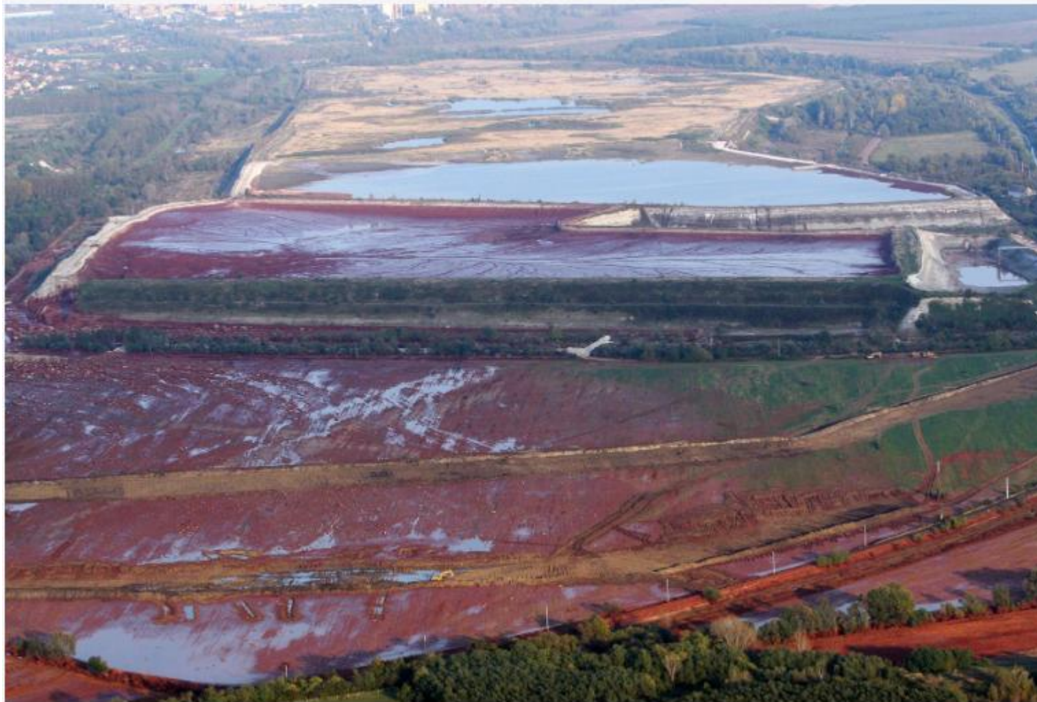
THE AJKA TAILINGS DAM FAILURE, 2010
