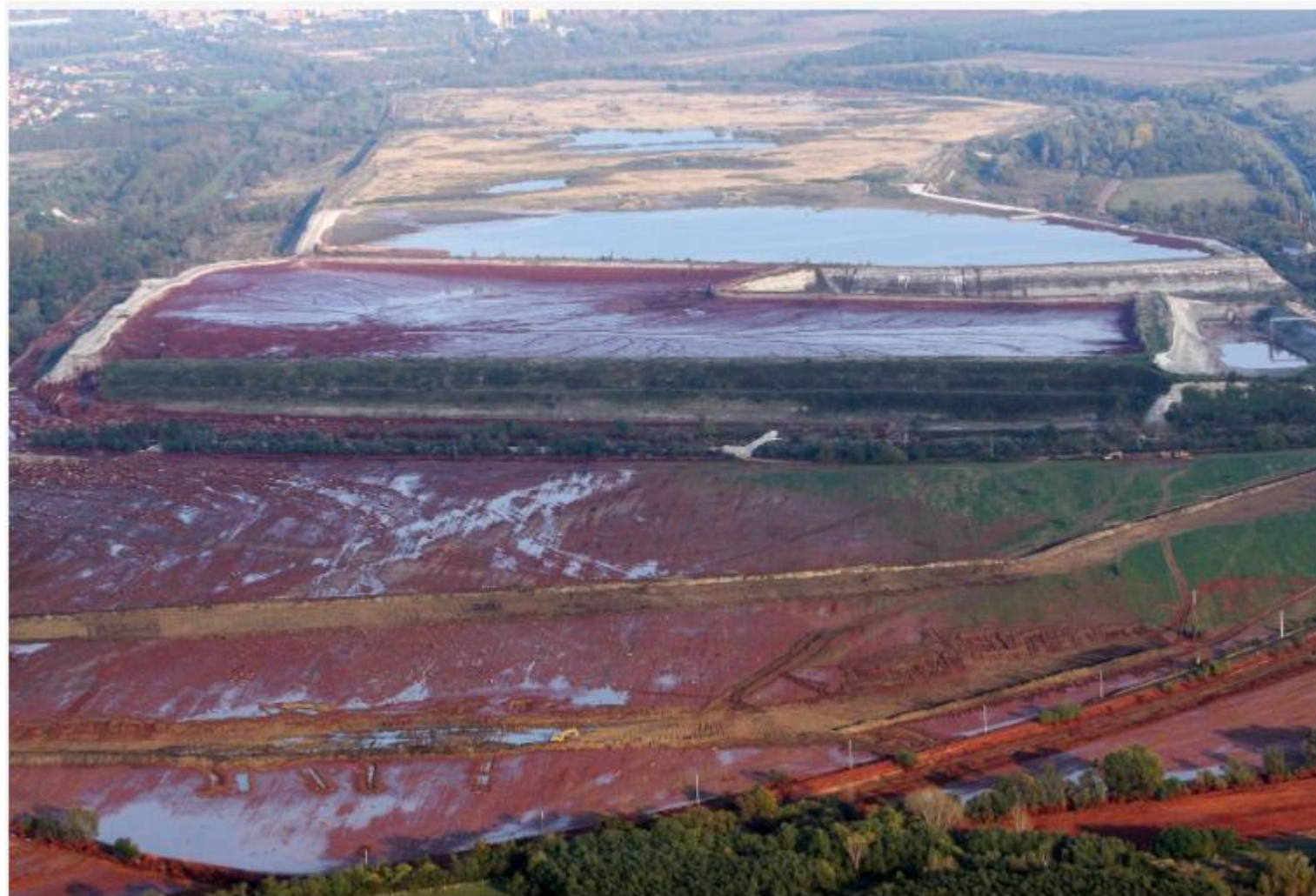
THE AJKA TAILINGS DAM FAILURE, 2010
